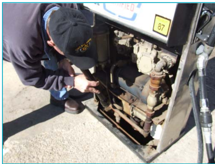
Tim Lutz, release prevention enforcement coordinator for BUSTR, inspects a gas pump for potential leaks.
