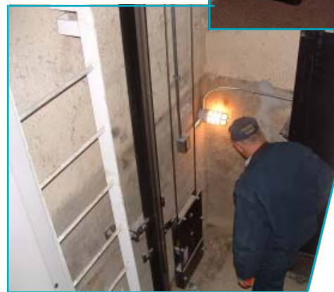
Elevator Inspector Doug Watkins conducts an inspection.
