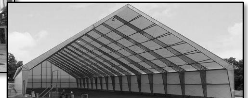
Membrane-Covered Frame Structure
