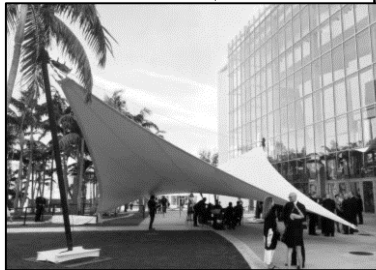
Membrane-Covered Cable Structure
